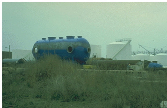
Above ground storage tanks
