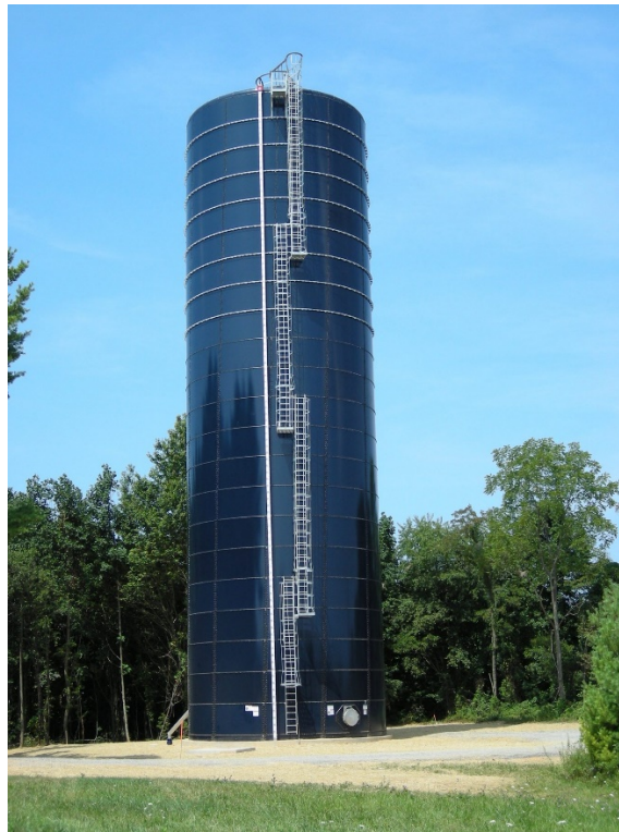
Aquastore Water Tower
